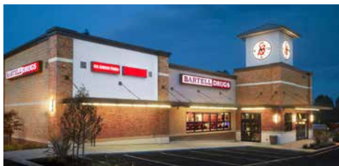
Bartell Drugs' Lynnwood, Washington location, which opened in May 2015, has 25 watt T8 linear fluorescent lamps installed to save energy and money.
