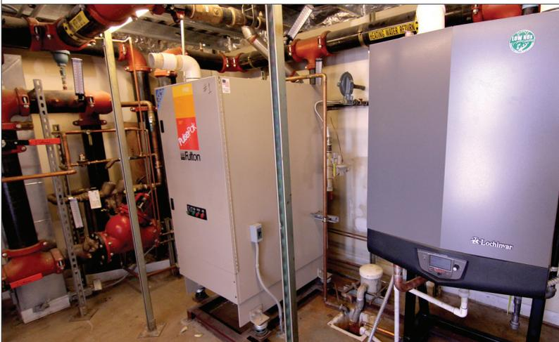
New energy-recovery unit and remote-access digital controls
