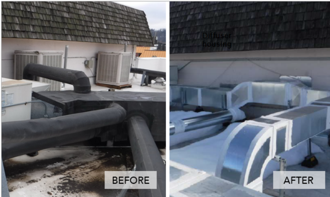
[FIGURE 8: EXAMPLE EXTERIOR DUCT SEALING]
